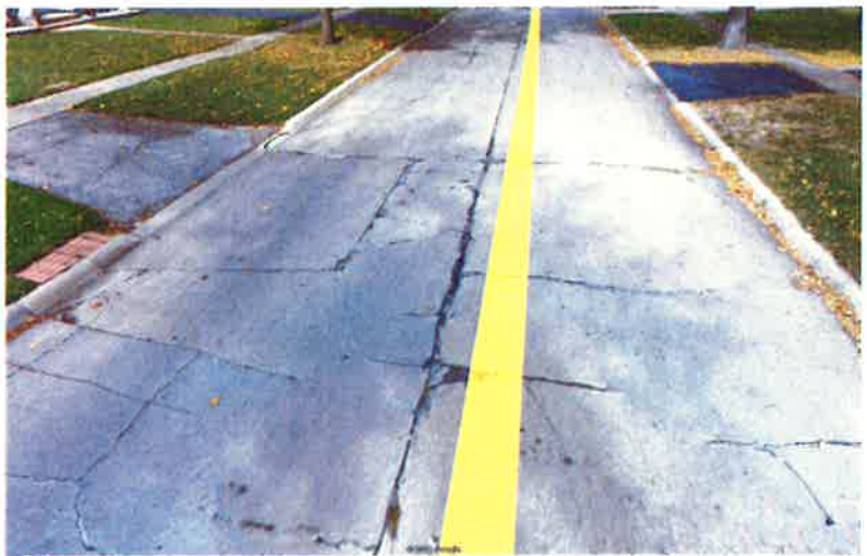
Photo 1 - Typical Concrete street in NW section
