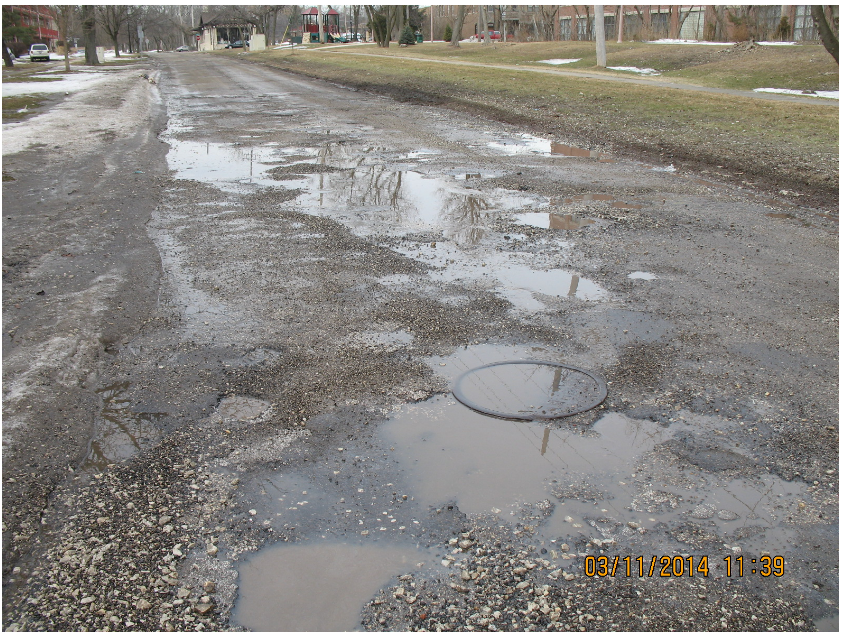
Park Blvd. – Villa to East End
