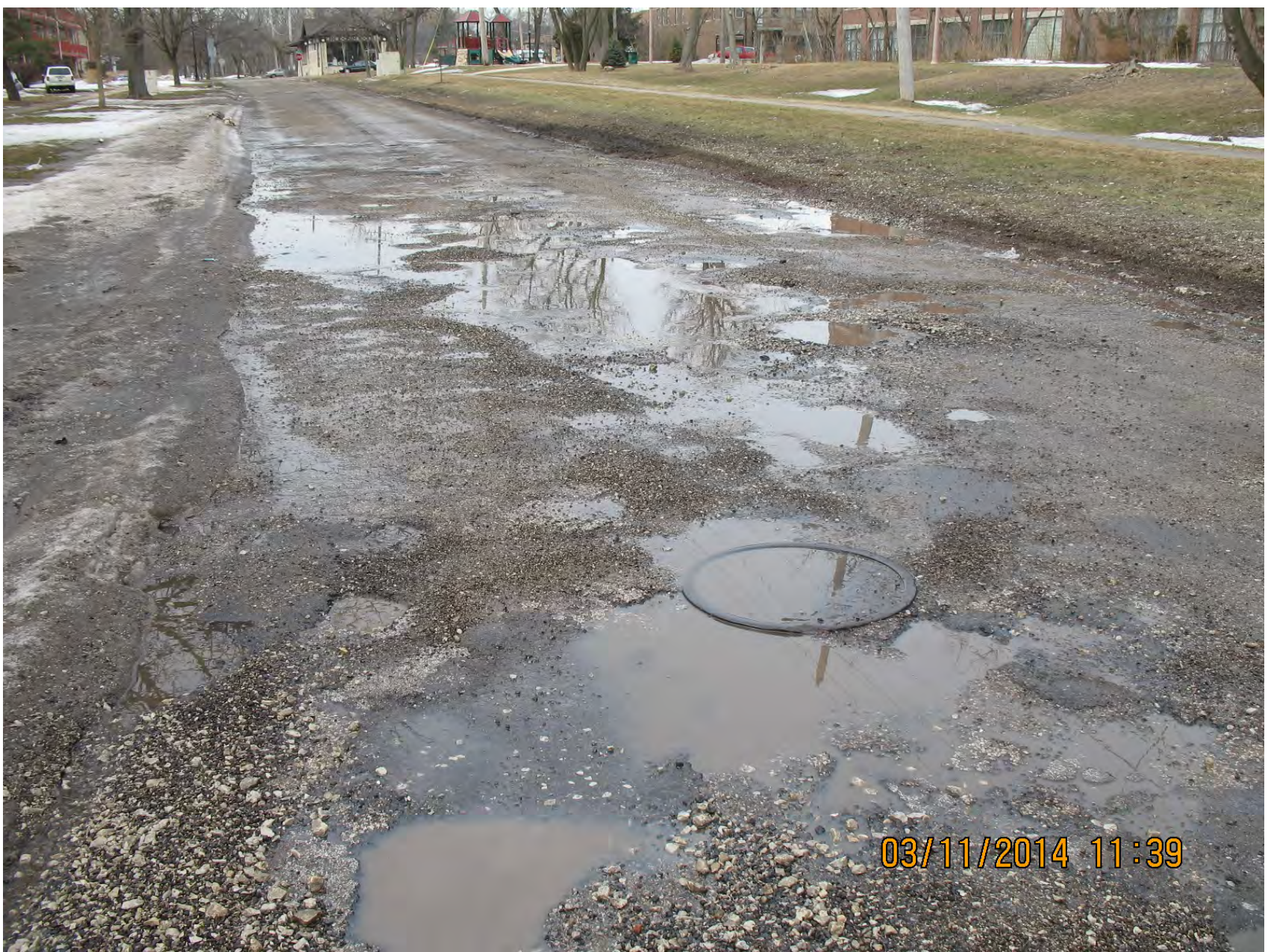
Park Blvd. – Villa to East End
