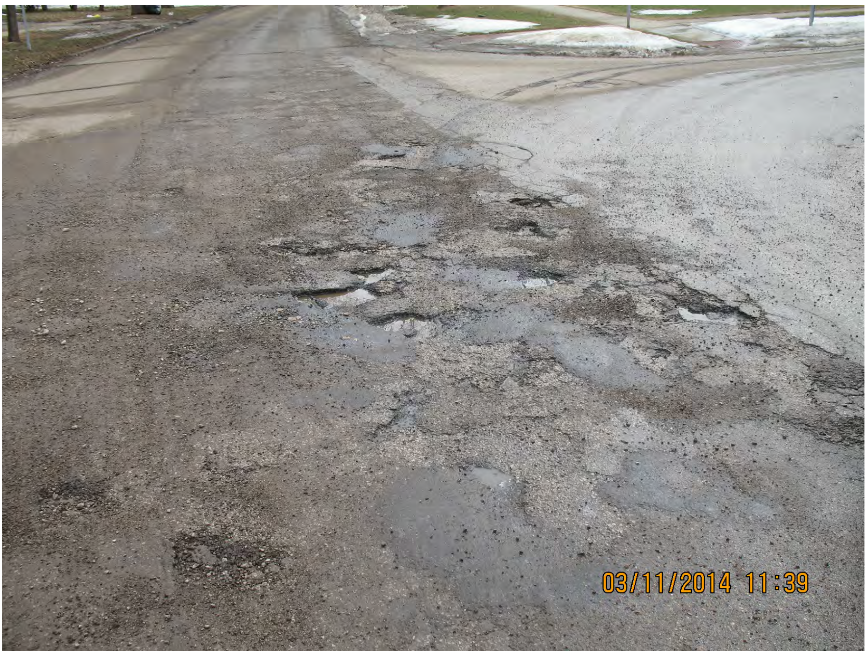
Park Blvd. – Villa to East End
