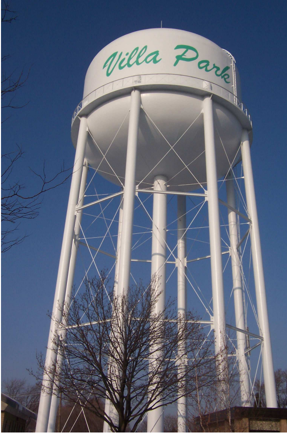
Villa Park Water Tower: Plymouth and Princeton
