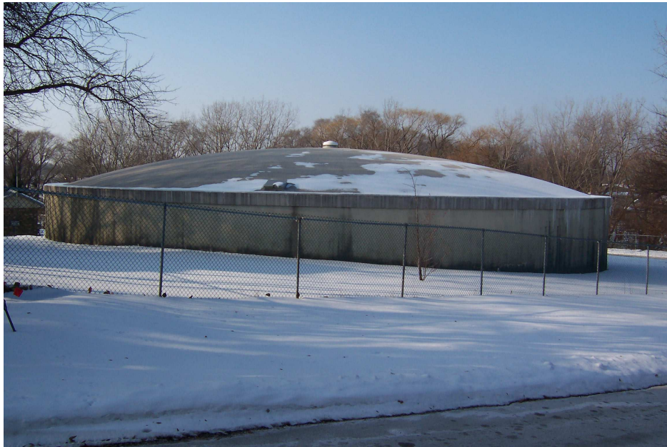
Cornell Reservoir: 2,000,000 gallons
