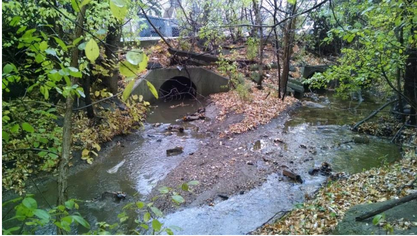
Storm Sewer Outfall
