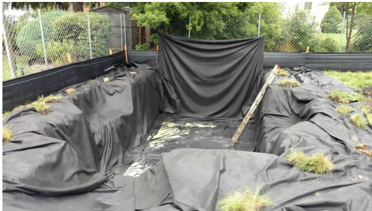
Example of BMP and sediment and erosion control
