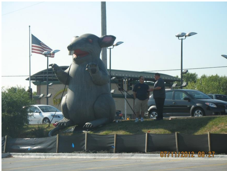
Example of Perimeter Silt Fence
