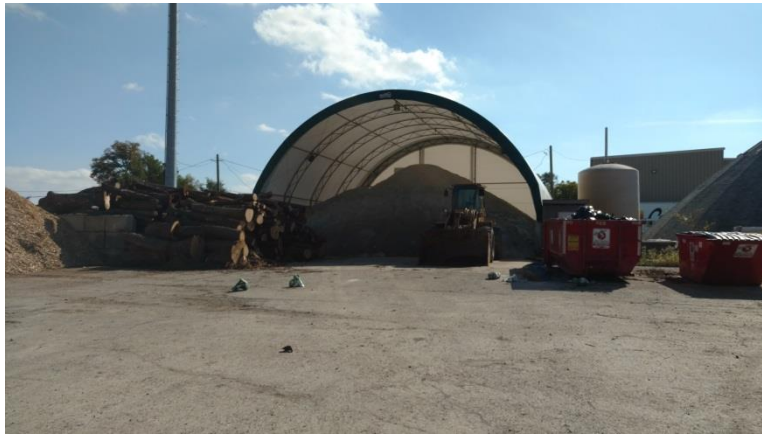
Village of Villa Park Salt Storage
