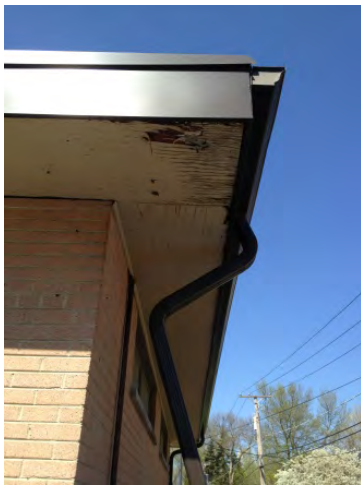
Soffit / Downspout at NE Corner
