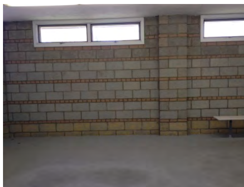
Men's Locker Room
