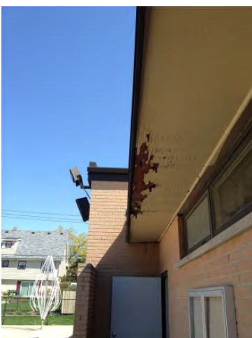
Soffit at West
