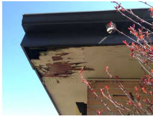
Soffit at SW Corner
