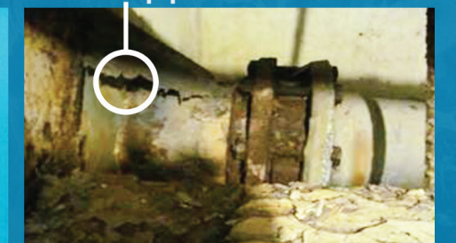
Corroded pipe
